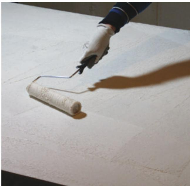
Photo 1. Applying RoomDamp2 constrained-layer damping compound to the back of sheathing to be sandwiched between sheathing layers.
